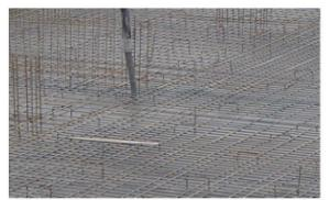
Fig. 1. Concreting in high density reinforcement
