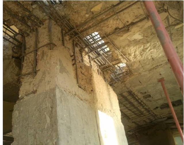
**Fig. (1) Bad quality concrete at upper part of column**
