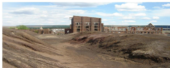
Fig. 1. General view of the industrial site of the AMP before elimination, 2009.
