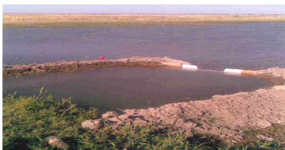
Fig. 3. Flooding of rice water flow check, check across the threshold of the spillway
