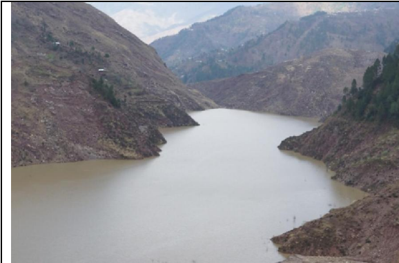
Figure 5. In February 2010, Karli lake breach out that resulted activation of landslide
