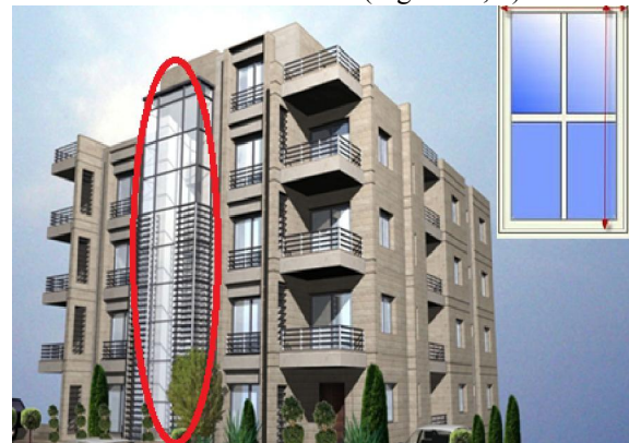
Fig. 1. The current building.
