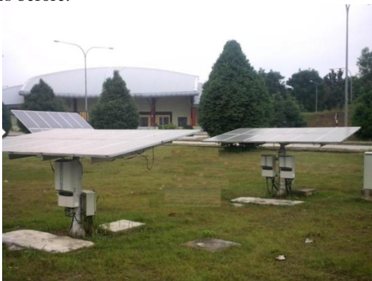
Figure 1. Fix flat photovoltaic in UPM site.
