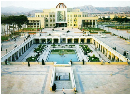
Figure 7: central courtyard of Khavaran Cultural Center with a view angle less than 9 degrees
