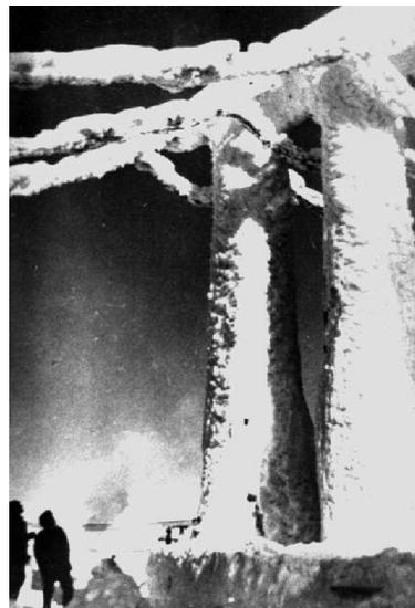
**Figure 1. Condition of a transmission line after a snow storm in Pavlodar oblast**
