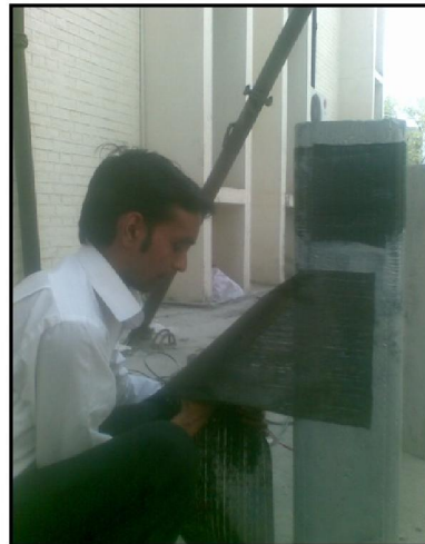
Fig.6 CFRP wrapping on concrete columns
