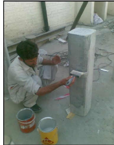
Fig.5 Application of epoxy resin on concrete column for CFRP confinement
