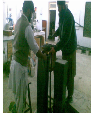
Fig.3 Casting of RC concrete columns
