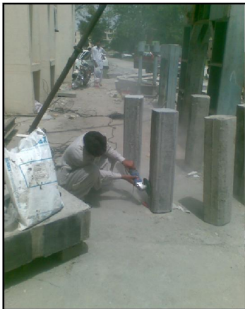
Fig.4 Preparation of concrete columns for CFRP confinement
