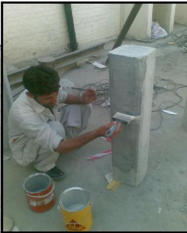
**Fig.6** Application of epoxy on concrete column for CFRP confinement
