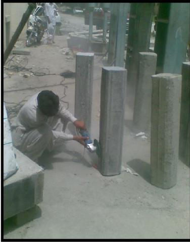
**Fig.5** Preparation of columns for confinement of CFRP wrap
