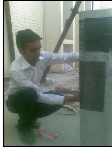
**Fig.7** CFRP wrapping on concrete column
