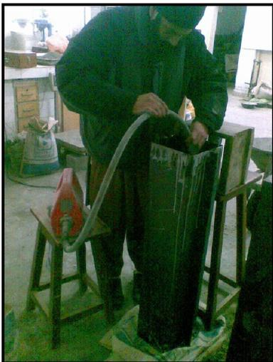
**Fig.3** Application of vibration to concrete through internal poker vibrator
