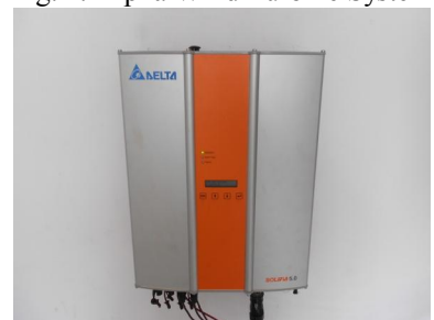
Fig. 3. SOLIVIA 5.0 Solar Inverter
