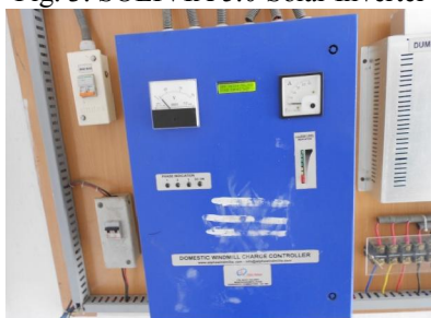
Fig. 4. Wind Mill Charge Controller
