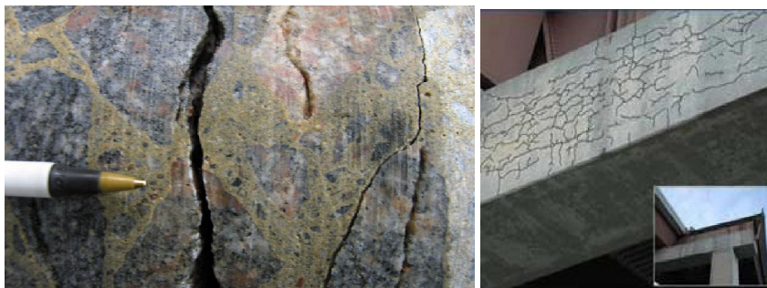
Figure 1- Samples of Cracking Caused by Alkali Reaction of Stones
