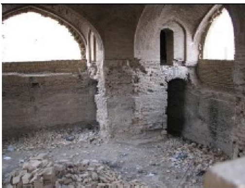
Figure 13 – Interior space of Haj Mirza water storage (Photo by Samira Tafazzol)
