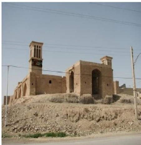
Figure 14 - View of Belan water storage on the hill (Photo by Samira Tafazzol)
