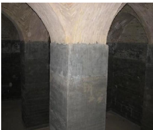
Figure 26 – Interior space of Oshkohran water storage (Photo by Samira Tafazzol)
