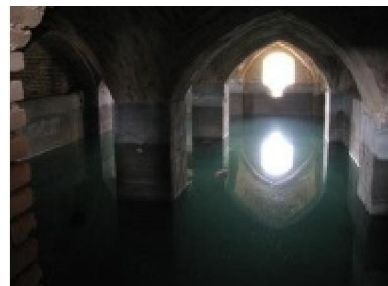
Figure 38- The interior space of Pechoviz water storage (Photo by Samira Tafazzol)
