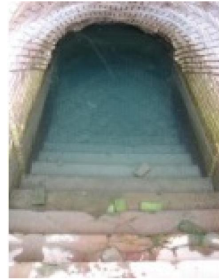
Figure 36- Pashir of Pechoviz water storage (Photo by Samira Tafazzol)
