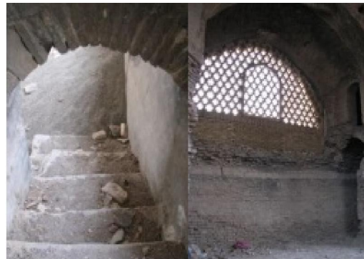
Figure 12 - stairways and gate of Haj Mirza water storage (Photo by Samira Tafazzol)
