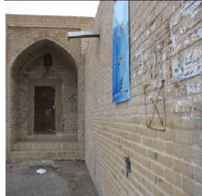
Figure 7 - The east side of Haji Muhammad Ja'far water storage (Photo by Samira Tafazzol)
