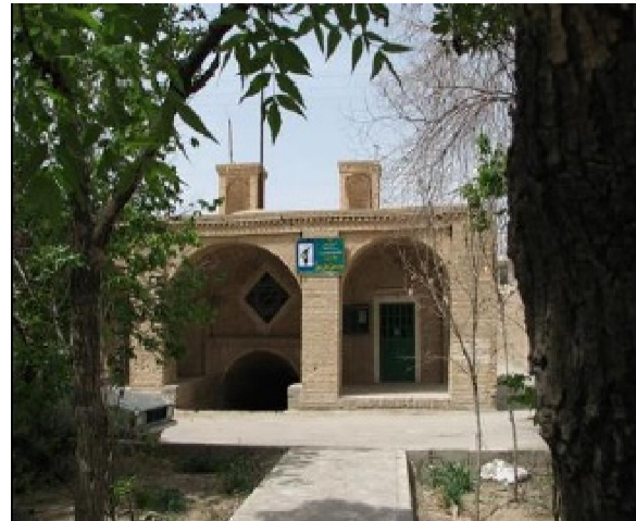
Figure 23 – Southern view of Oshkohran water storage (Photo by Samira Tafazzol)
