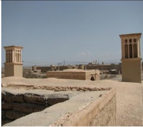
Figure 16 - View of roof and wind catcher of Belan water storage (Photo by Samira Tafazzol)
