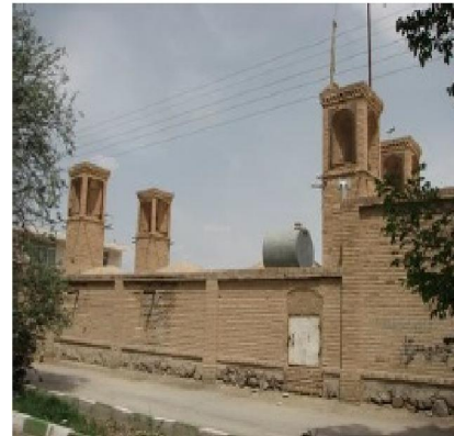
Figure 31- The tank and wind catchers of Oshkohran water storage (Photo by Samira Tafazzol)
