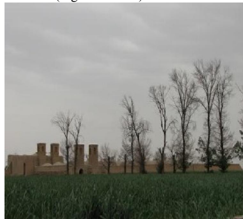
Figure 32- Perspective of Pechoviz water storage (Photo by Samira Tafazzol)
