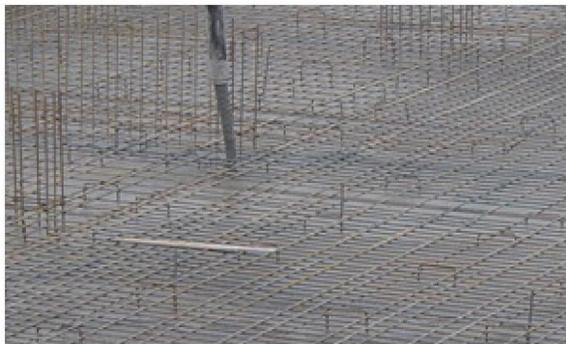
**Fig. 1. Concreting in high density reinforcement**
