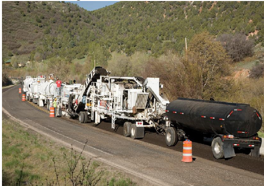
Figure 1: Cold In Place Recycling using Cold Recycling Train.
