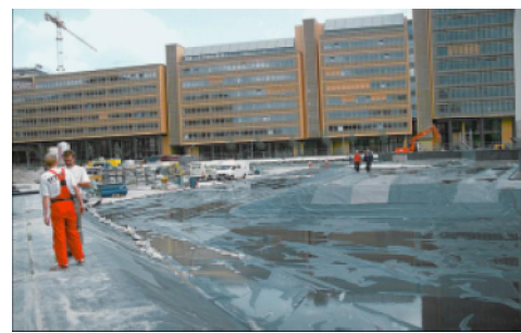
Figure 7: Constructed on top of a traffic tunnel, the biotope is lined with a geomembrane. (Atelier Dreiseitl, p111)
