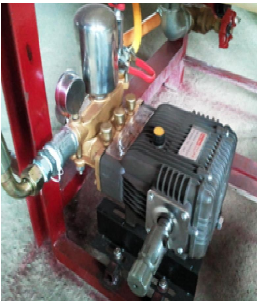
Figure 3. Water pump and main valves
