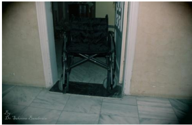
Fig. 3. Available space for the movement of the chair is not flexible enough for the passage of the chair easily by threshold and increase the difficulty of Use
