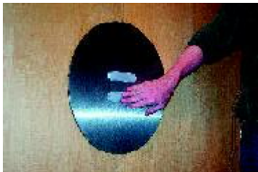
Fig. 4. The absence of detectable information makes these elevator call buttons difficult for first time users with reduced vision to recognize. (Rudolph et al., 2001 )
