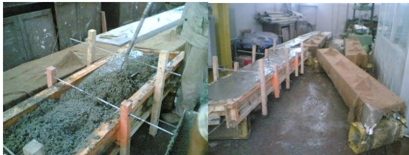
Fig. 5: Preparation and curing of composite decks
