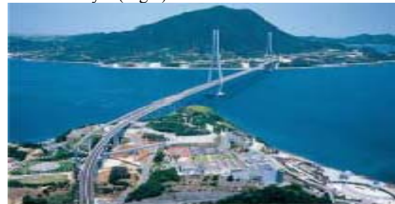
Fig. 4. Tataru Cable-Stayed Bridge
