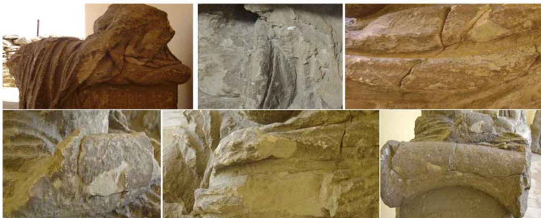
Fig. (2) Details of deterioration phenomena of the statues as surfaces degradation, crystallization of soluble salts, dark layers on the surfaces, vertical and horizontal deep cracks, erosion by wind effect and missing parts.
